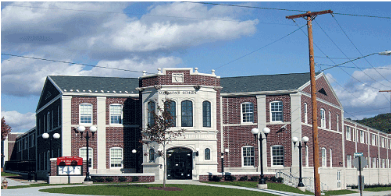
Figure 4: Modular School in Reading, Pennsylvania
