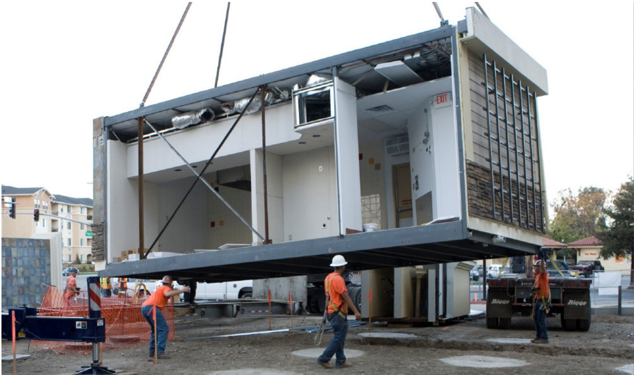
Figure 6: Modular being installed, lifted from above, all interior finishes and fixtures completed.
