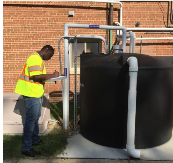
BMP Inspection, Fire Station 206
