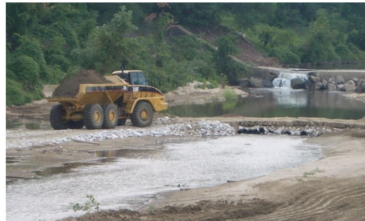
Channel maintenance, Cameron Run
