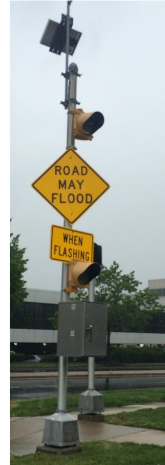
Flood warning sign and lights
