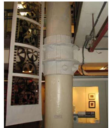
Column collars supporting the mezzanine level
